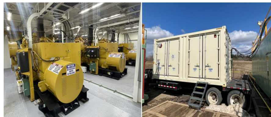
Figure 23: Natural Gas Power Generation and ESS Container and Trailer.
